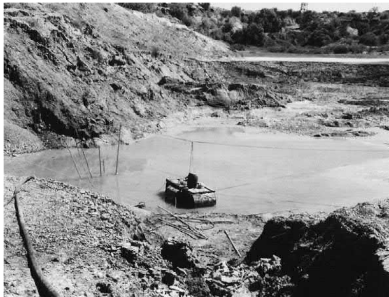
FIG. 6.9 Aftermath of the collapse of a tailings storage at a diamond mine into shallow underground workings. The level of the tailings before the collapse can be seen as a level surface in the background. The small pump barge is located over the site of the collapse.
