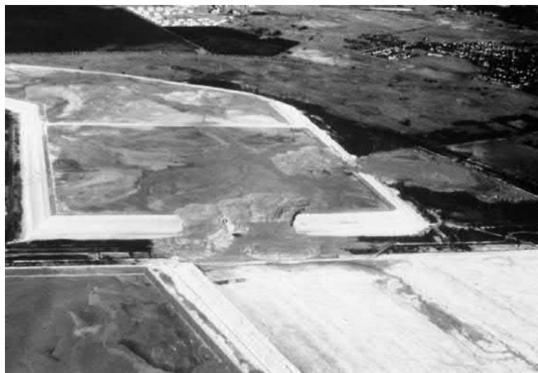
FIG. 6.12 Failures of a gold tailings storage at Saaiploas mine that was being built at an excessive rate of rise. (Two failures are visible, side by side in the center of the photograph, and one in the center-right.)
