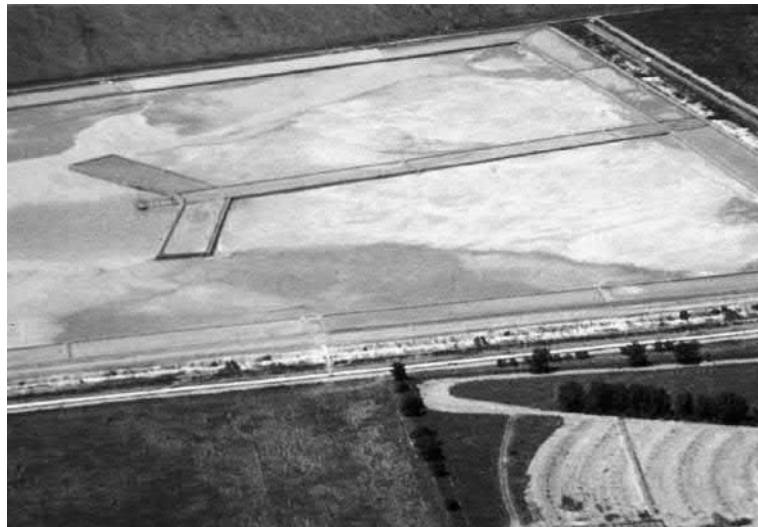
FIG. 6.7 A typical hydraulic fill tailings storage constructed by “beaching” toward a decant shaft.
